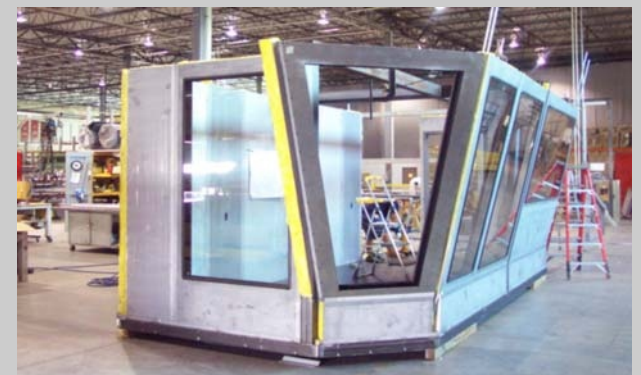
Custom Cantilevered Walls & Windows Being Assembled
