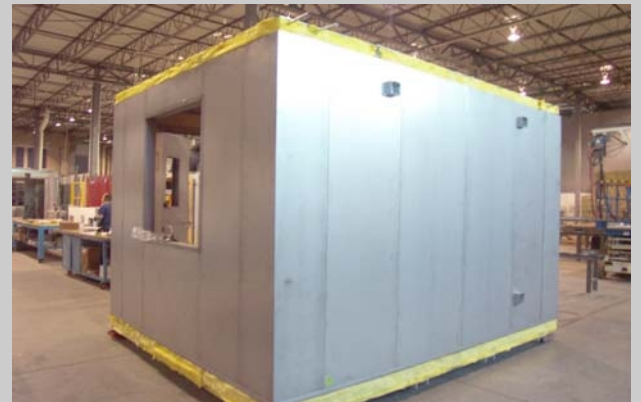
Assembled Structure Ready for Finishing Trim
