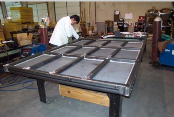
Custom Load Bearing Roof Section Being Fabricated
