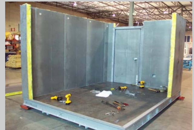
Modular Wall Panels Being Assembled Onto Base
