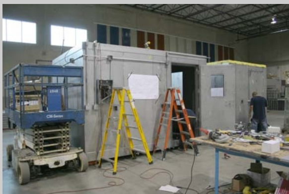
Electrical & Finish Work Being Completed
