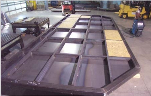
Custom Base Section Being Fabricated
